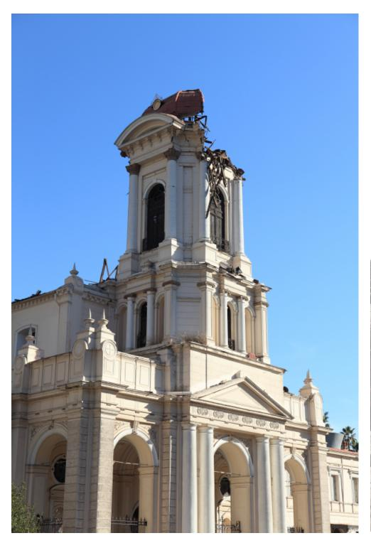
The church in the picture on the left, the *Iglesia de la Divina Providencia*, was built between 1881 and 1890 in Santiago. The top of the bell tower was destroyed by the earthquake in 2010.
